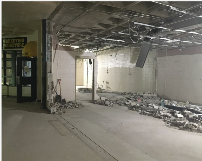
Bookstore & Classroom Wall Demolition
