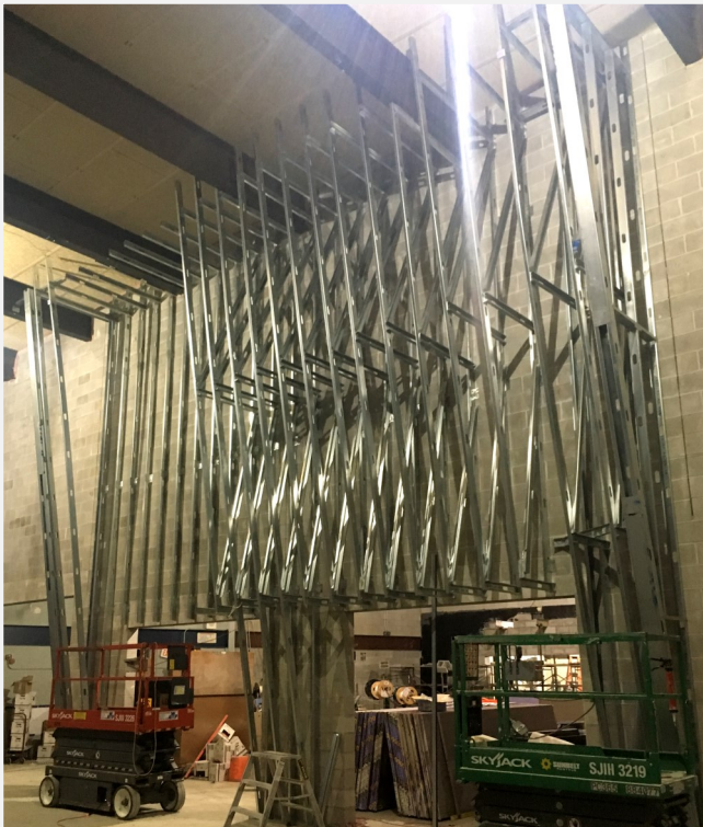
Wall Framing at Servery
