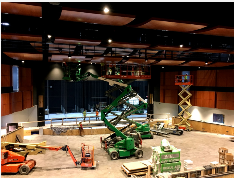
Auditorium Ceiling Cloud Installation
