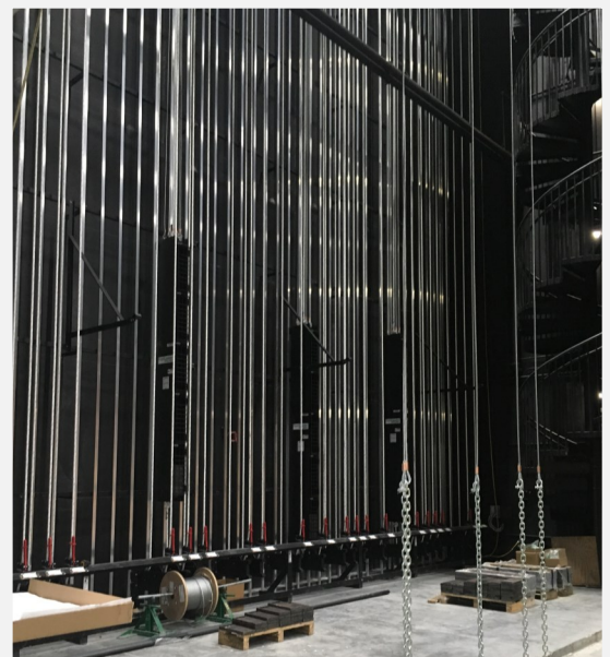
Auditorium Rigging Installation
