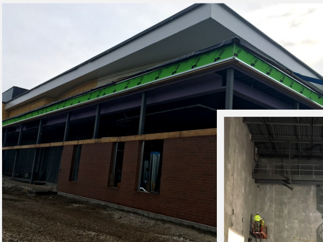
Auditorium Framing & Sheathing Progress
