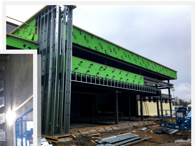
Gym Framing & Sheathing Progress
