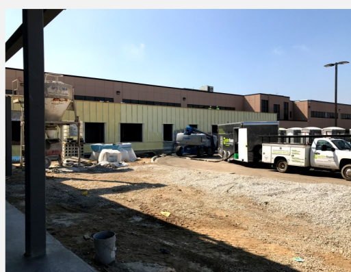
Offices Addition Spray Foam Installation
