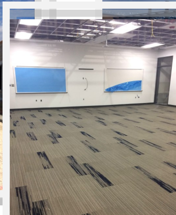
Remodeled Classroom Progress
