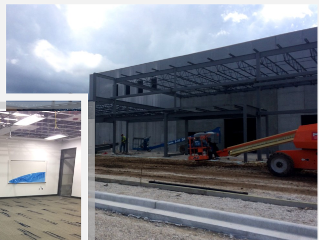
Erecting Steel at Gym Addition
