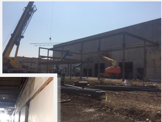
Erecting Steel at Gym Addition
