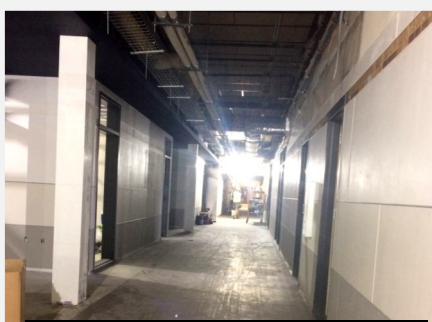
2nd Floor Corridor Wall Protection Panels
