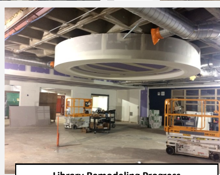
Library Remodeling Progress
