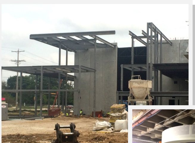
Auditorium Steel Erection Progress
