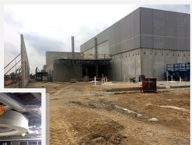
Gym Exterior Walls Progress
