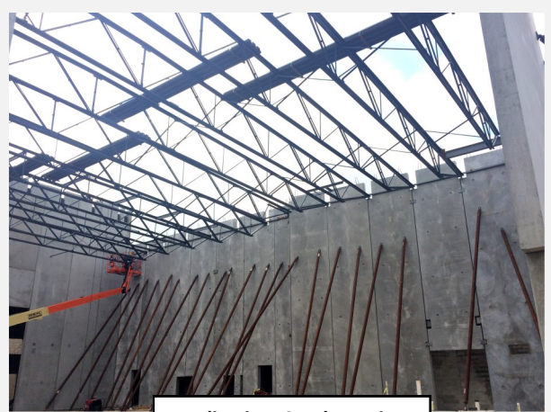
Auditorium Steel Erection
