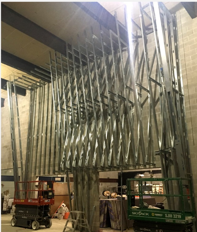
Wall Framing at Servery
