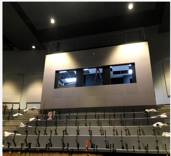
Auditorium Raised Seating Installation
