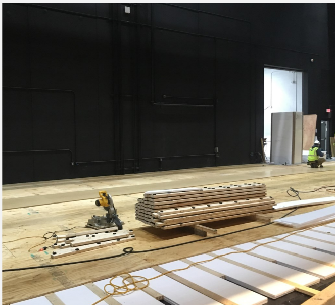
Auditorium Stage Floor Installation
