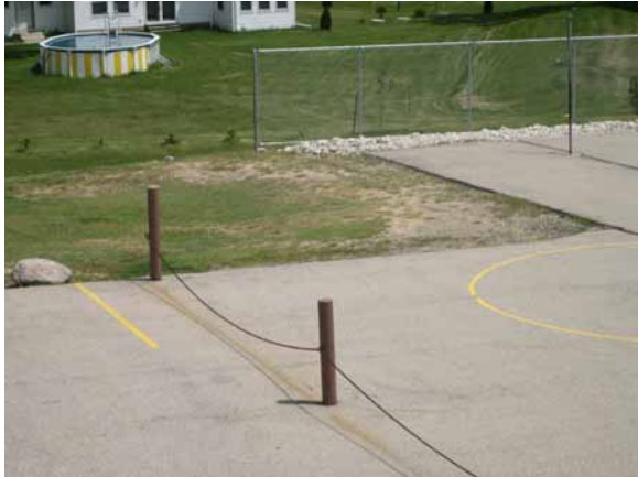
1.2 Asphalt paving at playground
