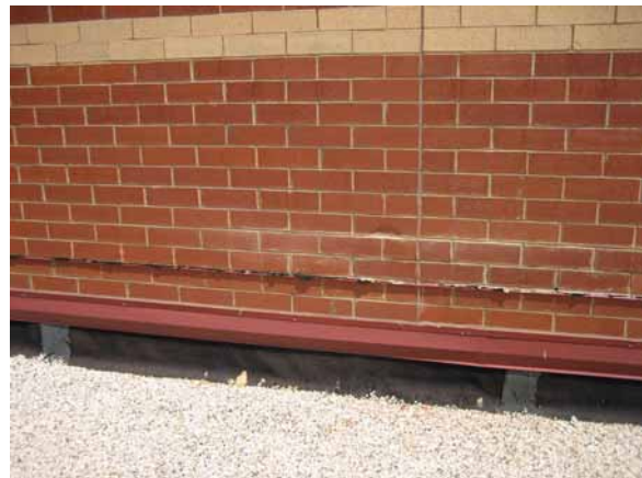
2.3 Brick repair at gym wall
