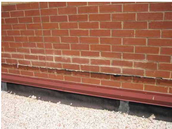
2.3 Brick repair at gym wall
